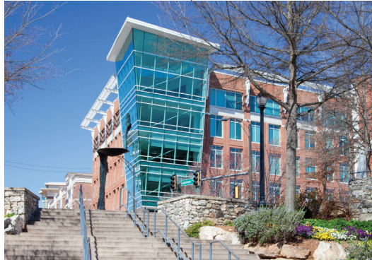
Above: The French tire maker Michelin was one of the first foreign companies to start a major manufacturing operation in South Carolina. Michelin currently operates plants in Anderson, Lexington, Columbia, Spartanburg, and Greenville, where Michelin North America is headquartered. In 2007, the company opened Michelin on Main in this futuristic building in downtown Greenville. This one-of-a-kind store sold Michelin collectibles and offered interactive activities until it closed in 2015.
